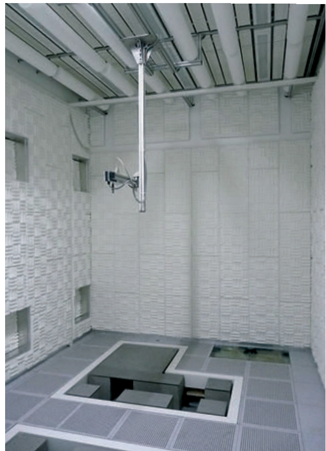
Experimentation room with 4.2 m clear room height and acoustic insulation materials (supplied and installed by Bilz). Source: Binnig and Rohrer Nanotechnology Center (IBM Research, Zurich).
